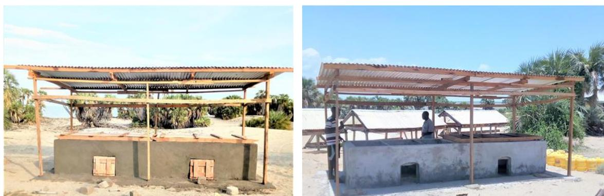
*Figure 5: complete Chorkor smoking kilns at Napeget (right) and Kalimapus (left) landing sites Lake Turkana*
